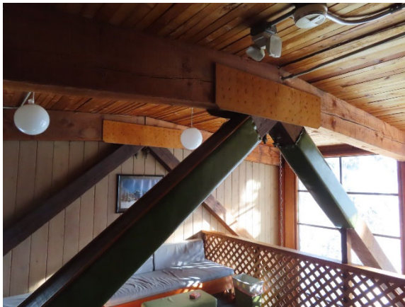
Timber Framing Supporting Roof
