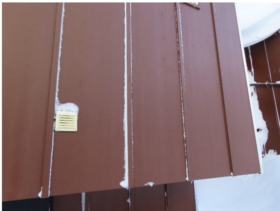
Area of New Fiber-Cement Siding
