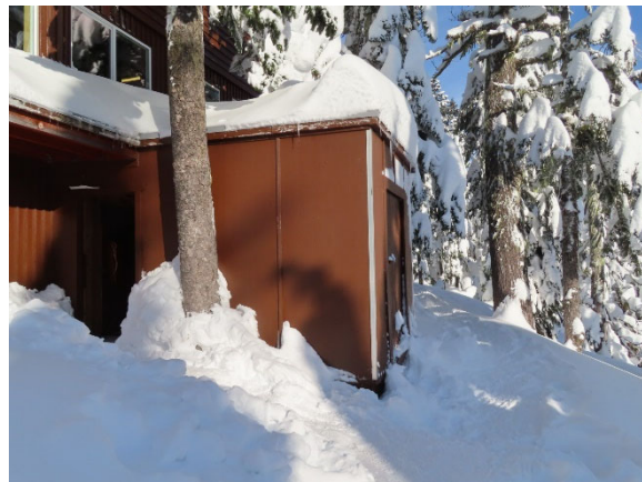
Exterior of Snow Tunnel
