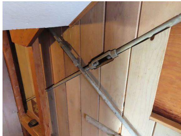
Steel Lateral Cross Bracing
