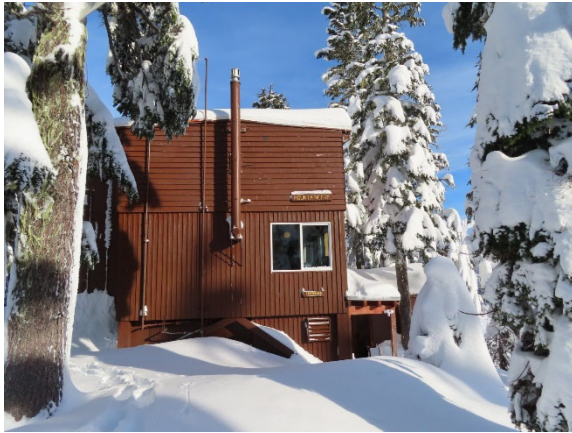
Southwest Side of the Building
