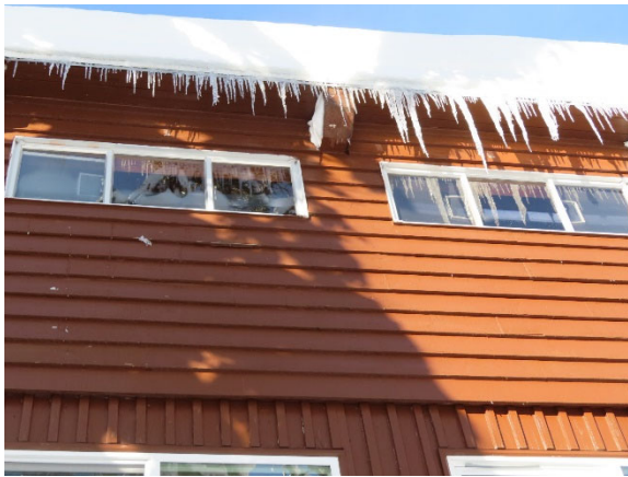
Close-up of Wood Lap Siding and Vinyl Windows
