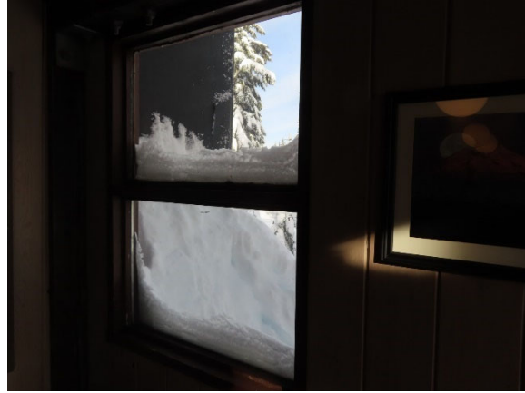
Typical Wood-Frame Window Viewed from the Interior
