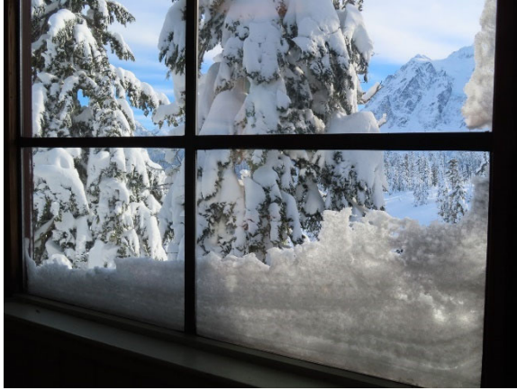
Typical Aluminum-Frame Window Viewed from the Interior
