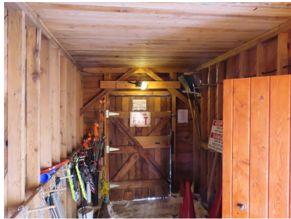
Interior of Snow Tunnel
