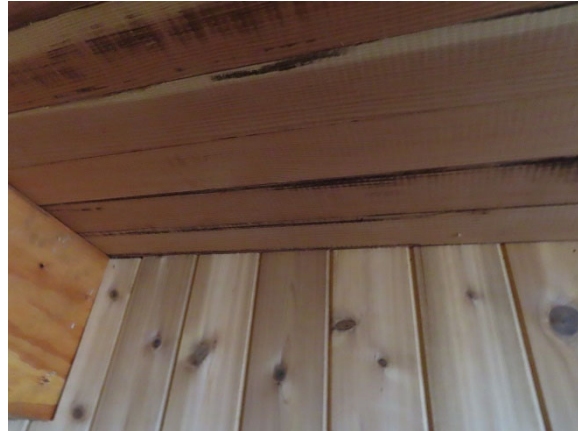
Wood Clad Ceiling and Walls on Third Floor
